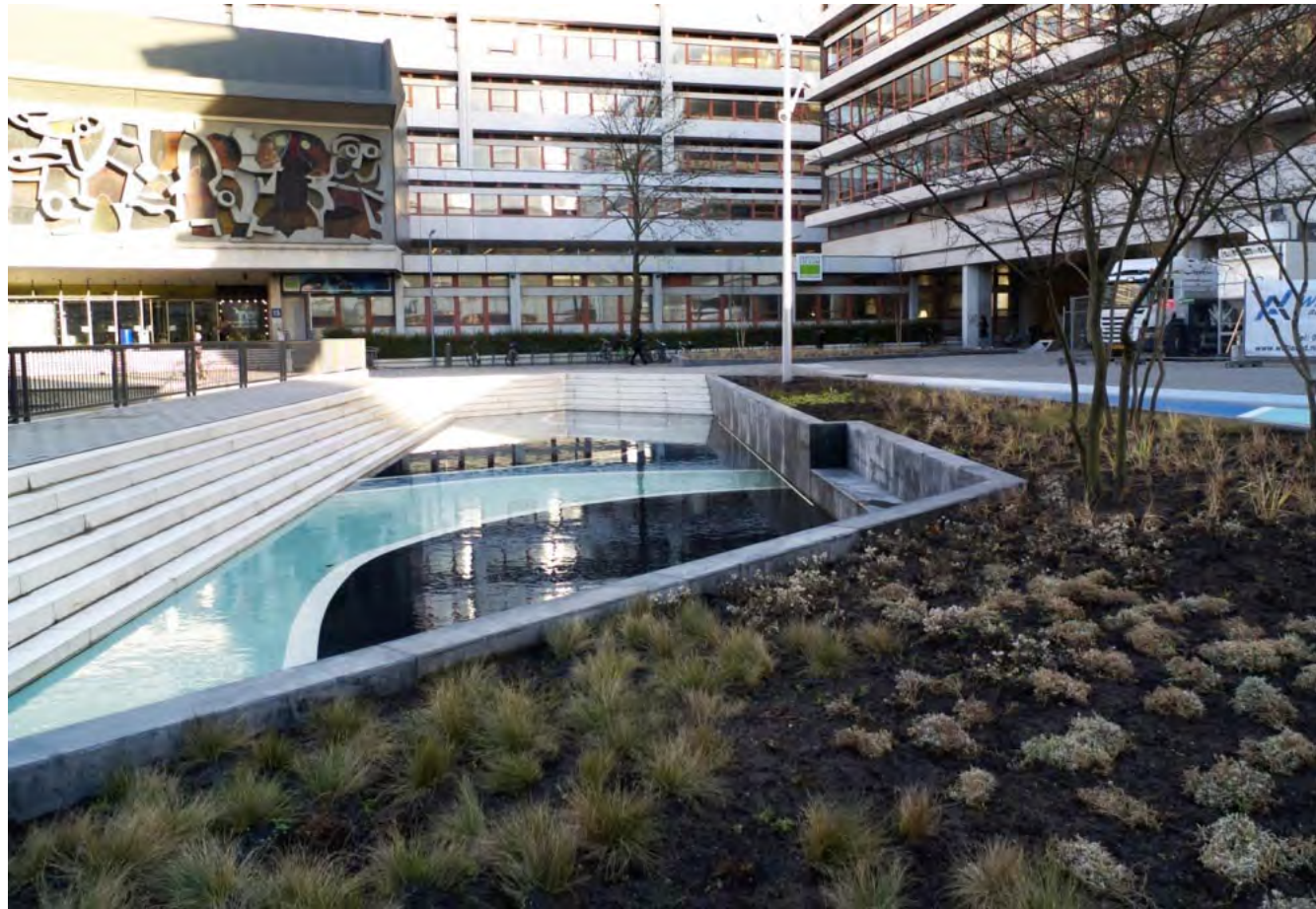
Water Square, De Urbanisten
