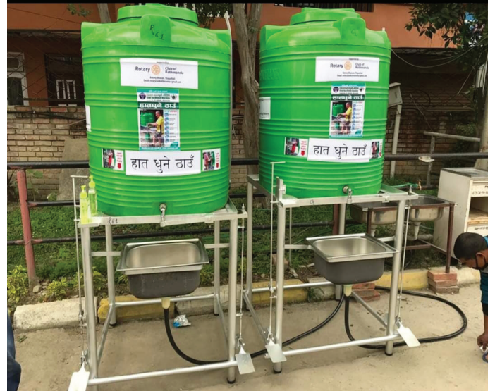
Dhulikhel Hospital hand washing units
